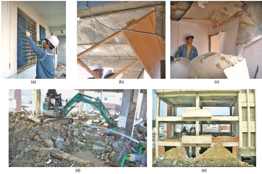
Photo 4A.1: Selective Demolition
