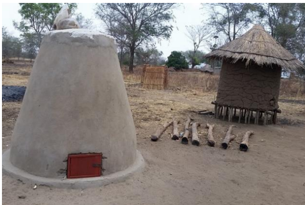
Picture 17 A concrete elephant safe food container constructed in a village close to Luambe National Park, Zambia. © E. Gross
