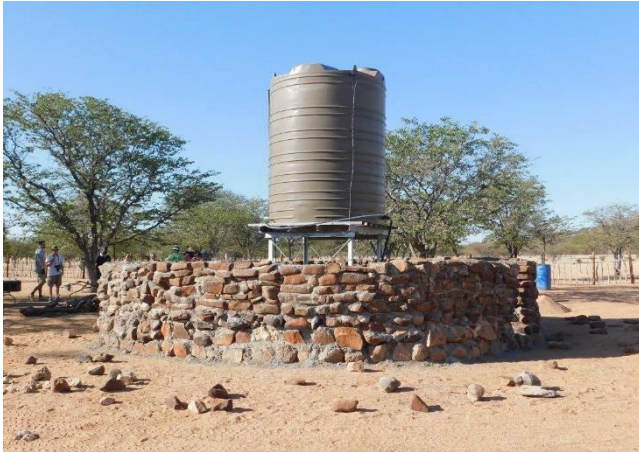
Picture 18 A water point secured by a stone and concrete wall in Namibia. © EHRA
