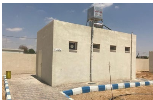
Figure 8: Accessible toilets at Salah Eddin Mosque, Mafraq.
