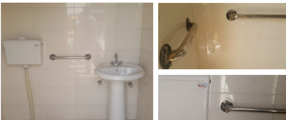
Figure 7: Accessible toilets at basic health units have been fitted with grabrails and an inside wash basin.
