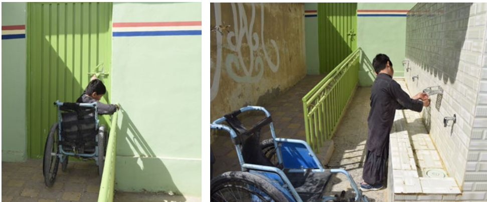
Figure 6: With the adjustments made, students using a wheelchair can now access toilets via the ramp and use handwashing facilities without assistance.
