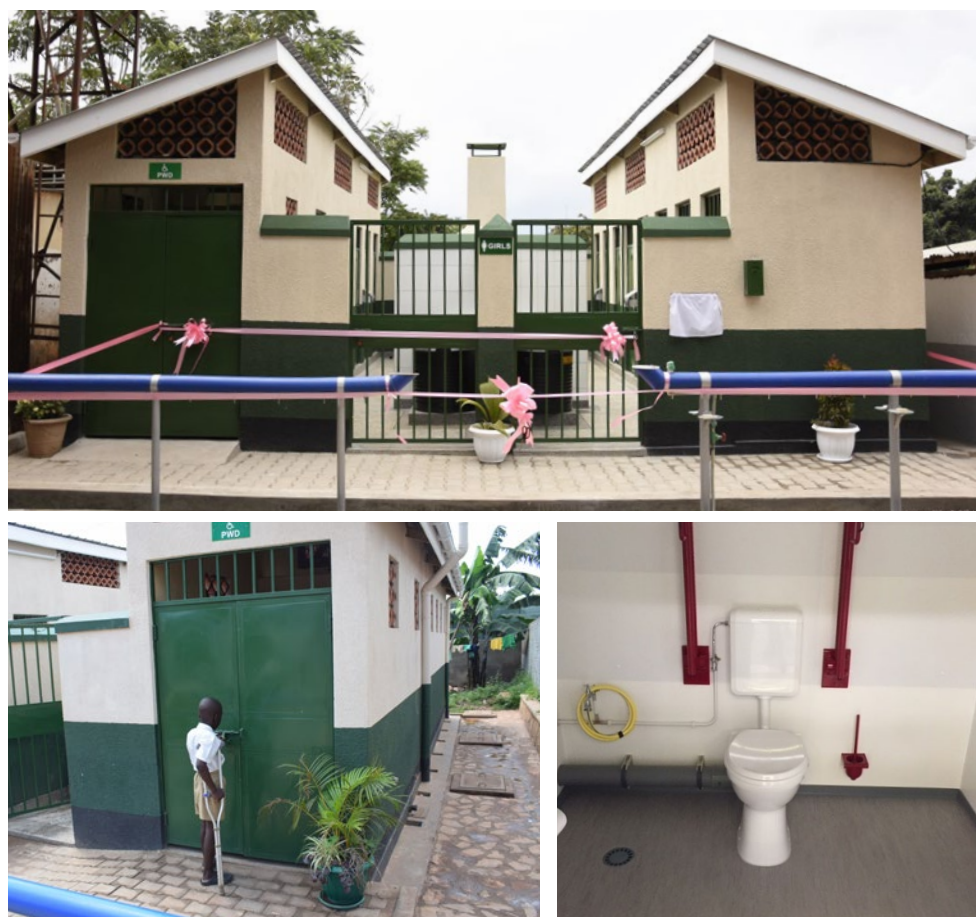
Figure 1: Toilet block with PWD cubicle in the girls' wing at St Peter's Primary School Nsambya, with WASHaLOT 3.0 group handwashing facilities in front.
