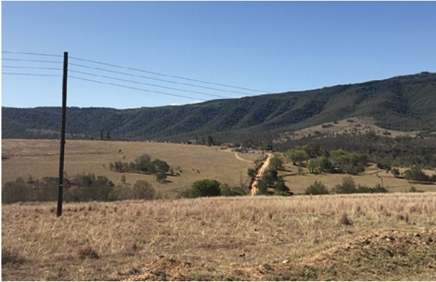
Figure 29: Distribution line connecting two sides of the village
