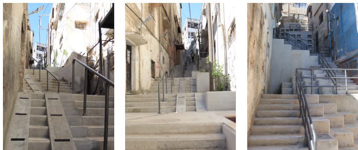
Fig 12: Construction progress from the Seventh Stair on Al-Quds Street
