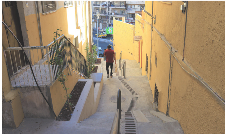
Fig 27: Small GI intervention - trenches implemented next to planters on Seventh Stair on Al-Quds Street, as a green stormwater solution
