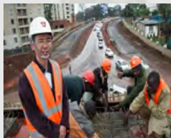
Chinese investment in Kenya to build a road
