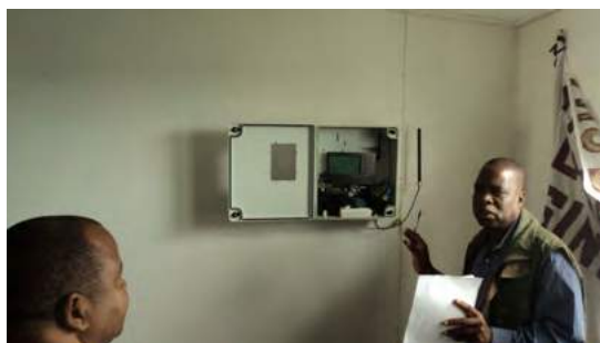
Equipments installation Source: Bank of Photos GIZ MZ
