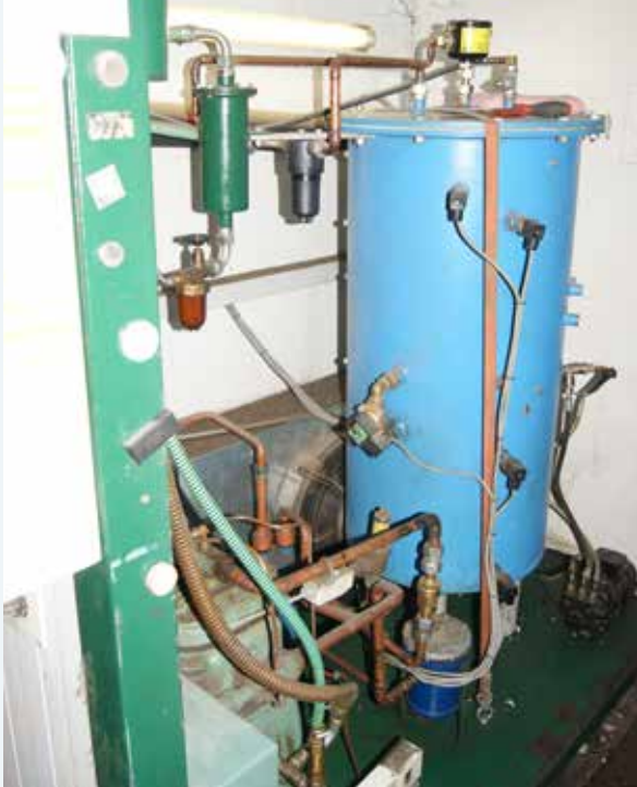
Separating refrigerant-oil mix
