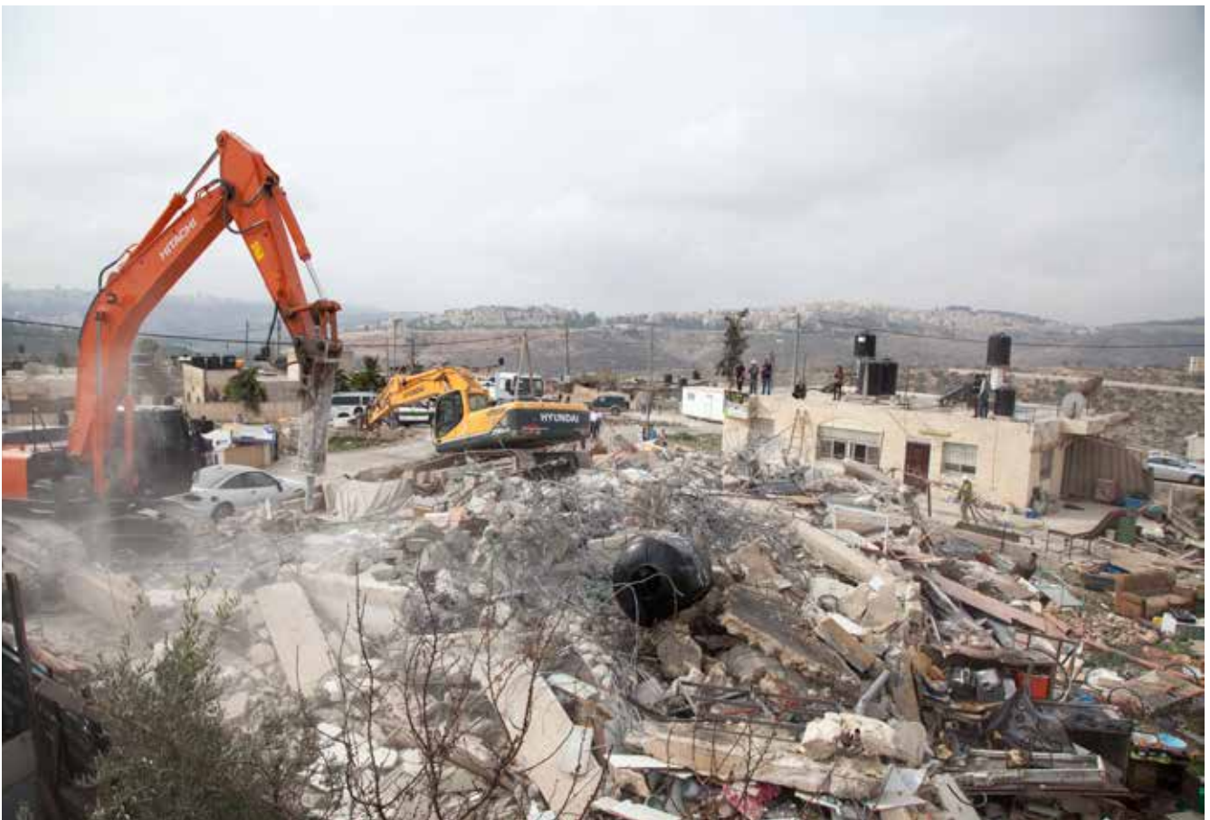
House Demolition Palestine 2016
