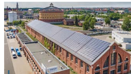
Sustainable energy supply systems on an existing building: The solar system on the historically listed "Kathedrale" has a nominal power of 260 kWp and yearly avoids approx. 170t of CO 2 . Source: LVV
