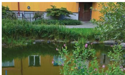
Pond in a residential area which also acts as storm water catchment. Source: Ulrika Pöppius
