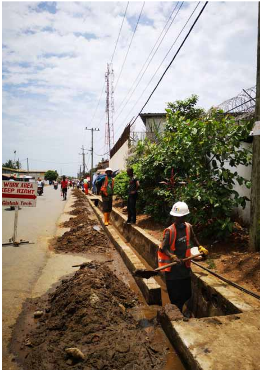
Routine road maintenance drainage cleaning.
