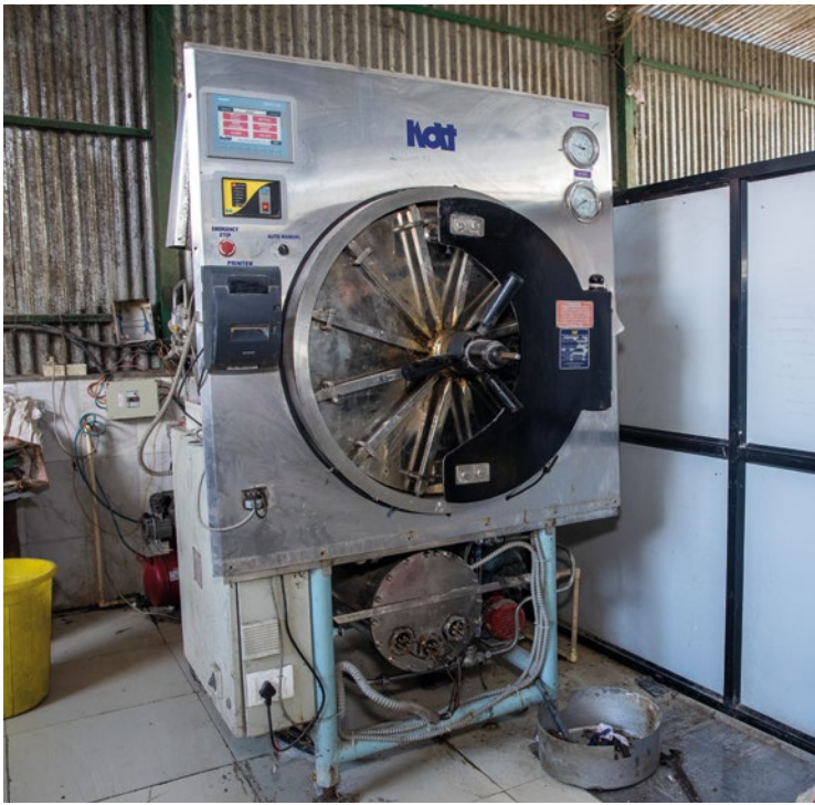
→ One of two autoclaves for treating healthcare waste at the Pokhara CTF
