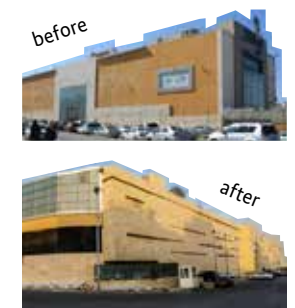
Fig. 7 Istiklal Mall in 2013 and 2014 before and after renovations
