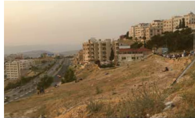
View onto Jordan Street, the Talit Al Wadi Restaurant, and a line of parked cars next to the brownfield
