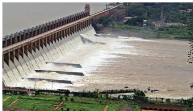
Dam Tungabhadra River, Hospet, Karnataka, India
