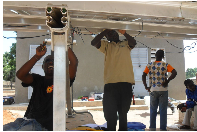
Ongoing works to install solar mini-grids, © by Ousmane Fall Sarr
