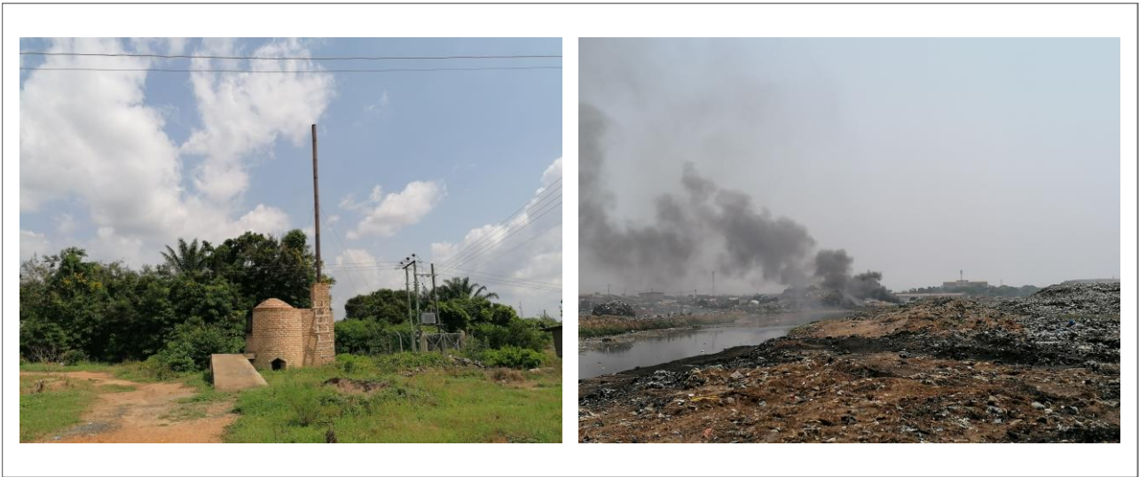
Figure 4-11: Incineration facility in Vume, Volta region (left), uncontrolled burning on the former scrapyards of Agbogbloshie
