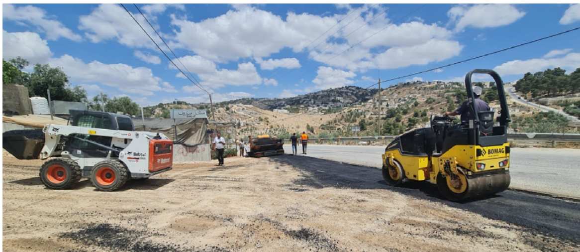
Surif Municipality constructing a new road
