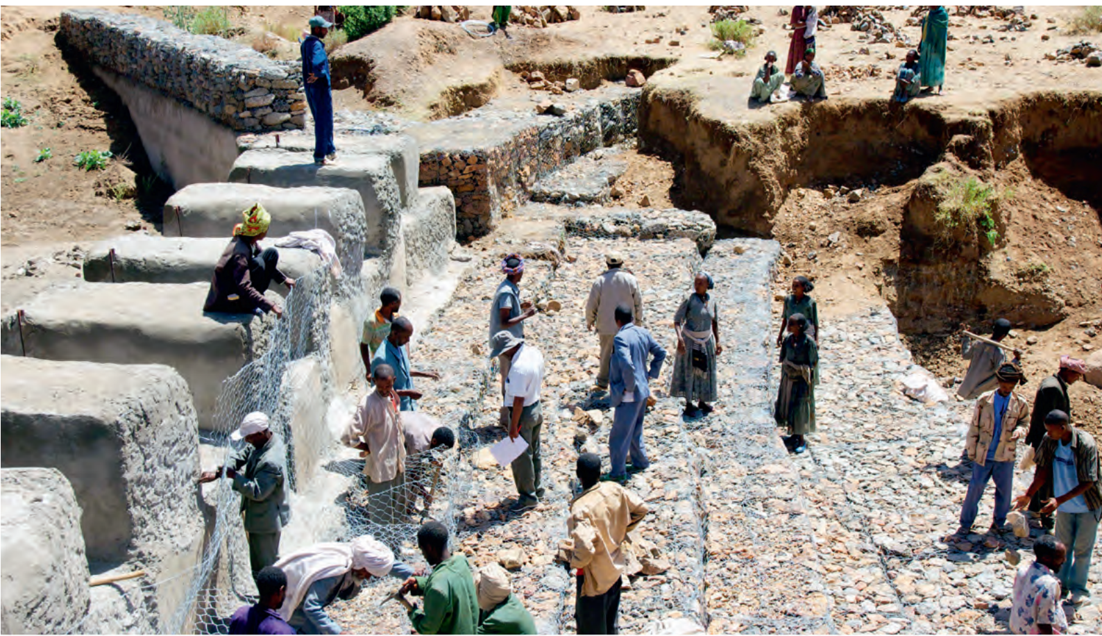
Sustainable Land Management Ethiopia | Smallholder groups combat soil loss and depletion by building terraces.
