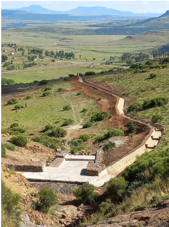
Diversion weir and canal
