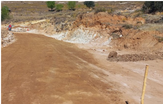
Road reshaping and stormwater management
