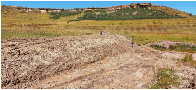
Raising of the small earth dam
